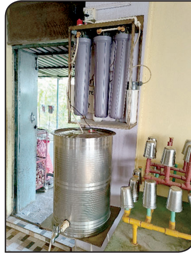
Vigyan ashram kitchen filter with UV tube fitment
